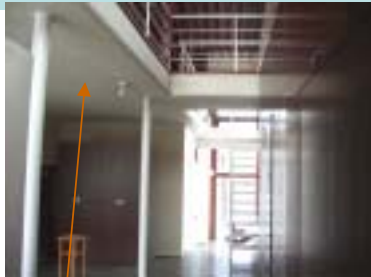
Plastering wall made from powder of Wakkanai Siliceous Shale
