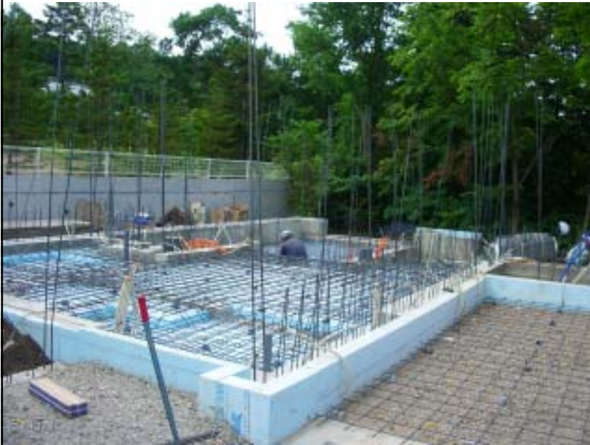
Building foundation is surrounded by Styrofoam
