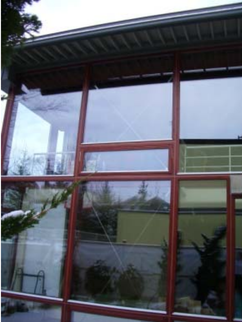
Southern glazing curtain wall construction
