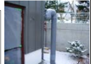
Heat and cool tube VP 200 mm \phi Depth=1.1m, Length=40m
