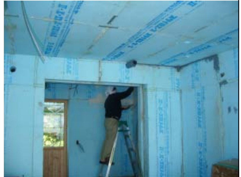
Inner walls of the garage are covered by Styrofoam
